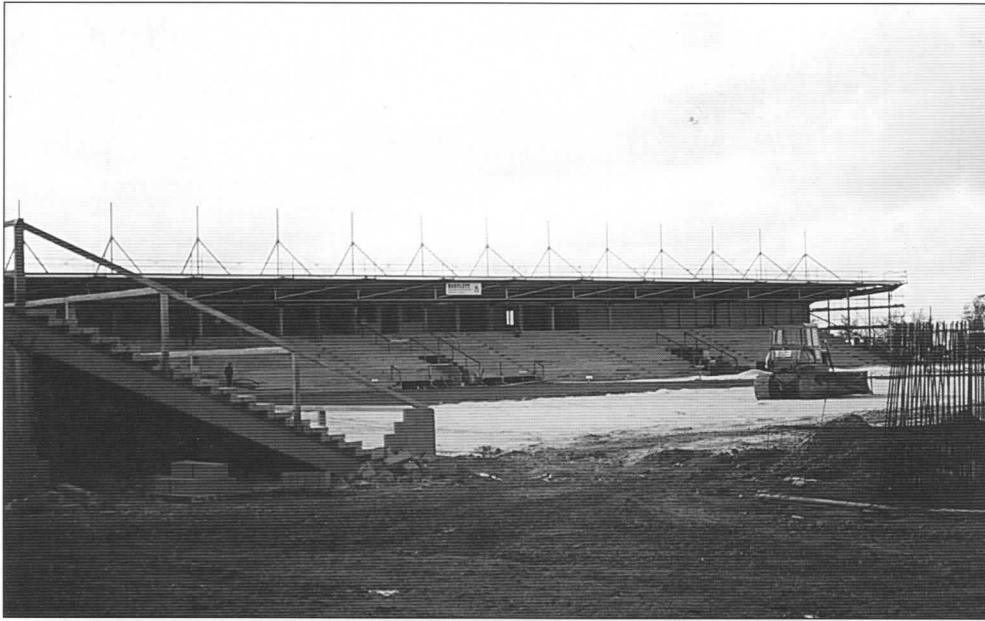
The Huish Park ground under construction.
