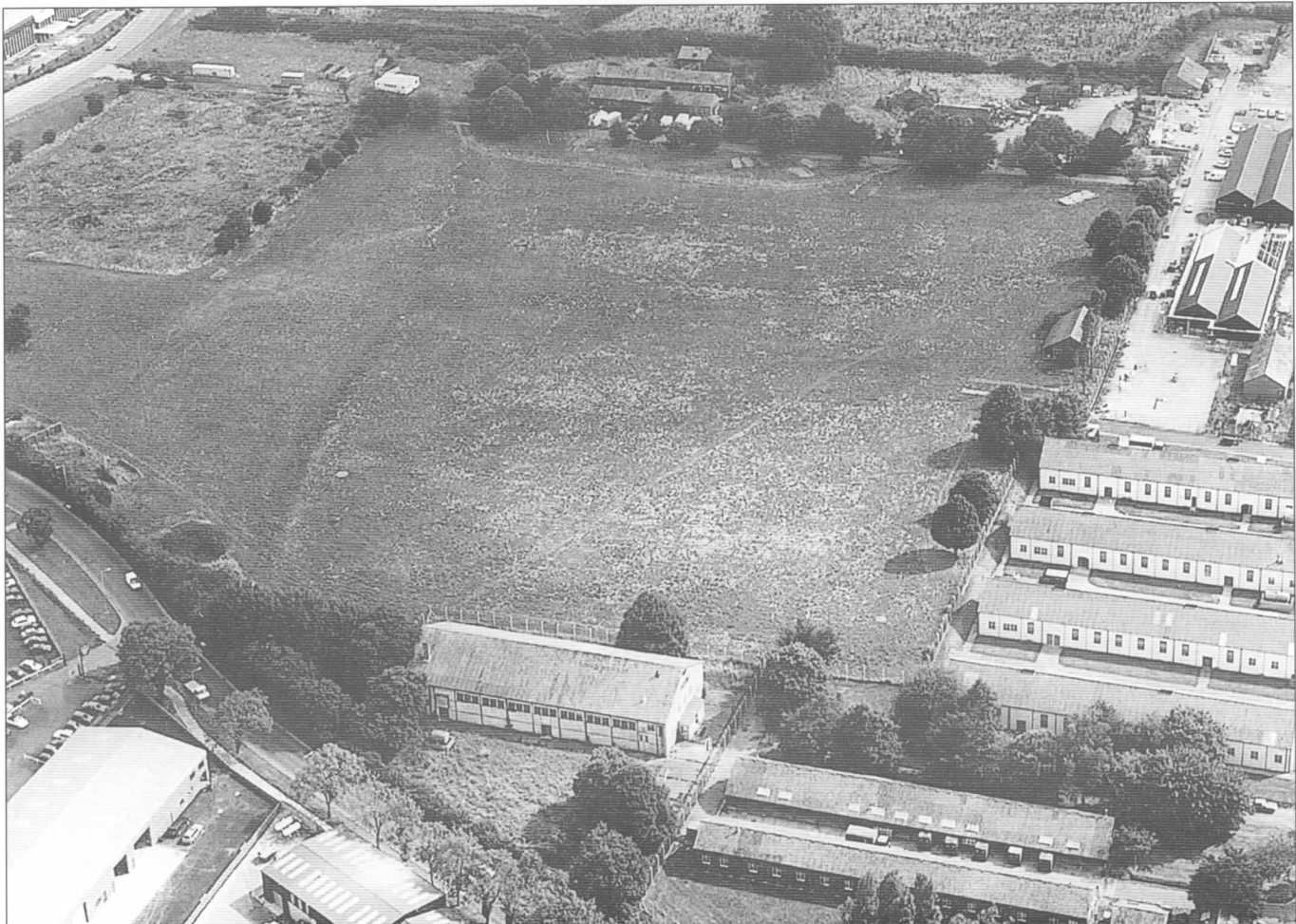
An aerial shot of the Huish Park ground at Houndstone before work began.
