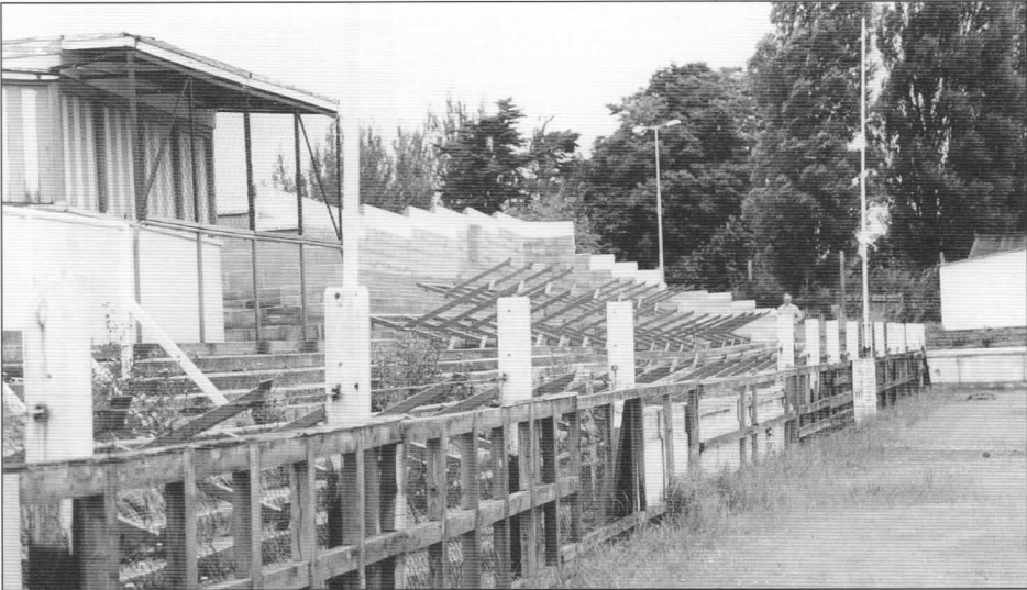
The demolition of Huish during the summer of 1990
