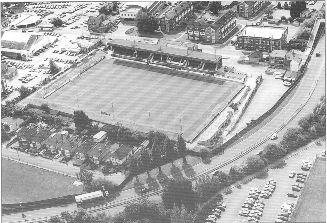
An aerial shot of the Huish ground before demolition.
